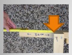
The next step are the two legs 190cm from behind the target. You place the legs 35 cm from the top of the front frame with one screw 5x70.
