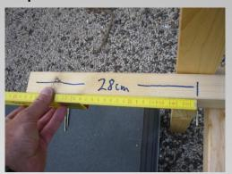
Turn a screw 5x70 by 28 cm of the end in the middle of the frond leg.
